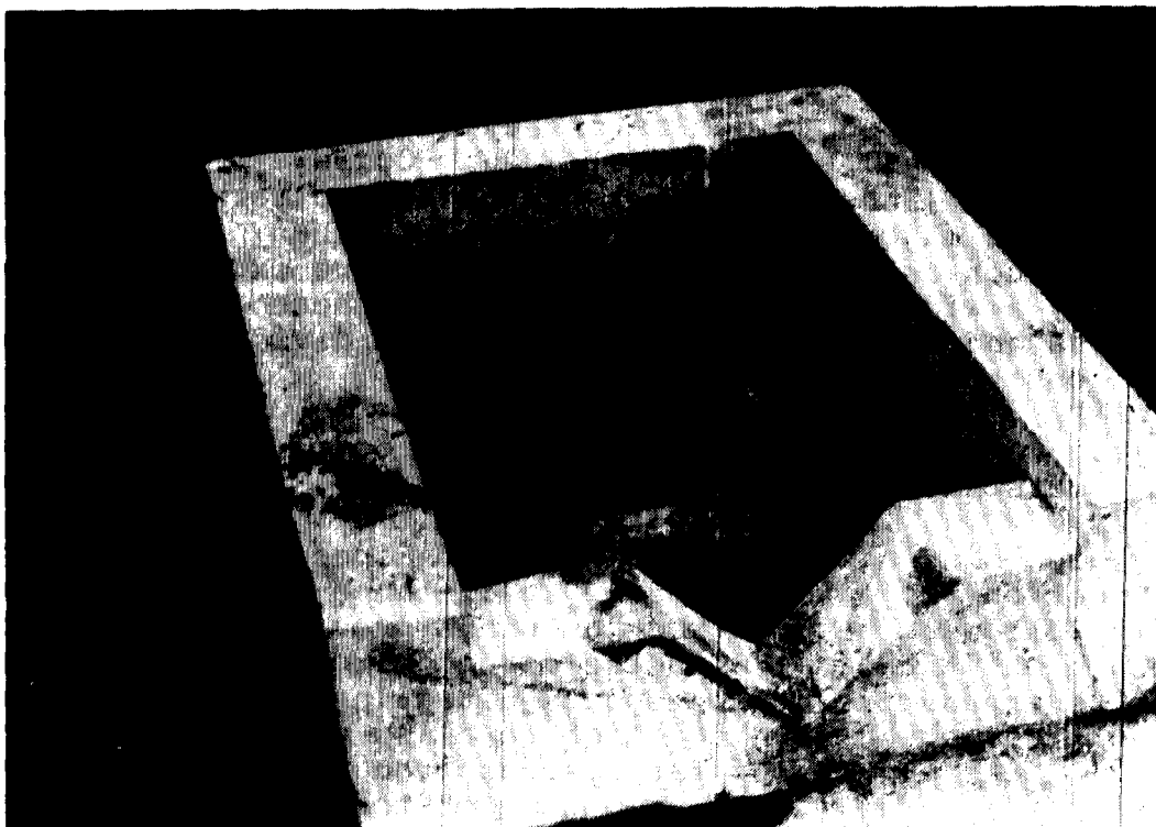
Turnout box and valve for underground pipe allow farmer to regulate water flow
