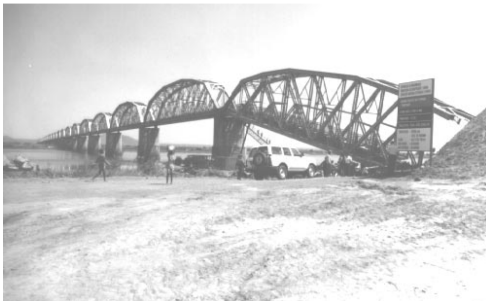
Figure 7: Railroad Bridge in Mozambique That Was Repaired With Child Survival Funding
