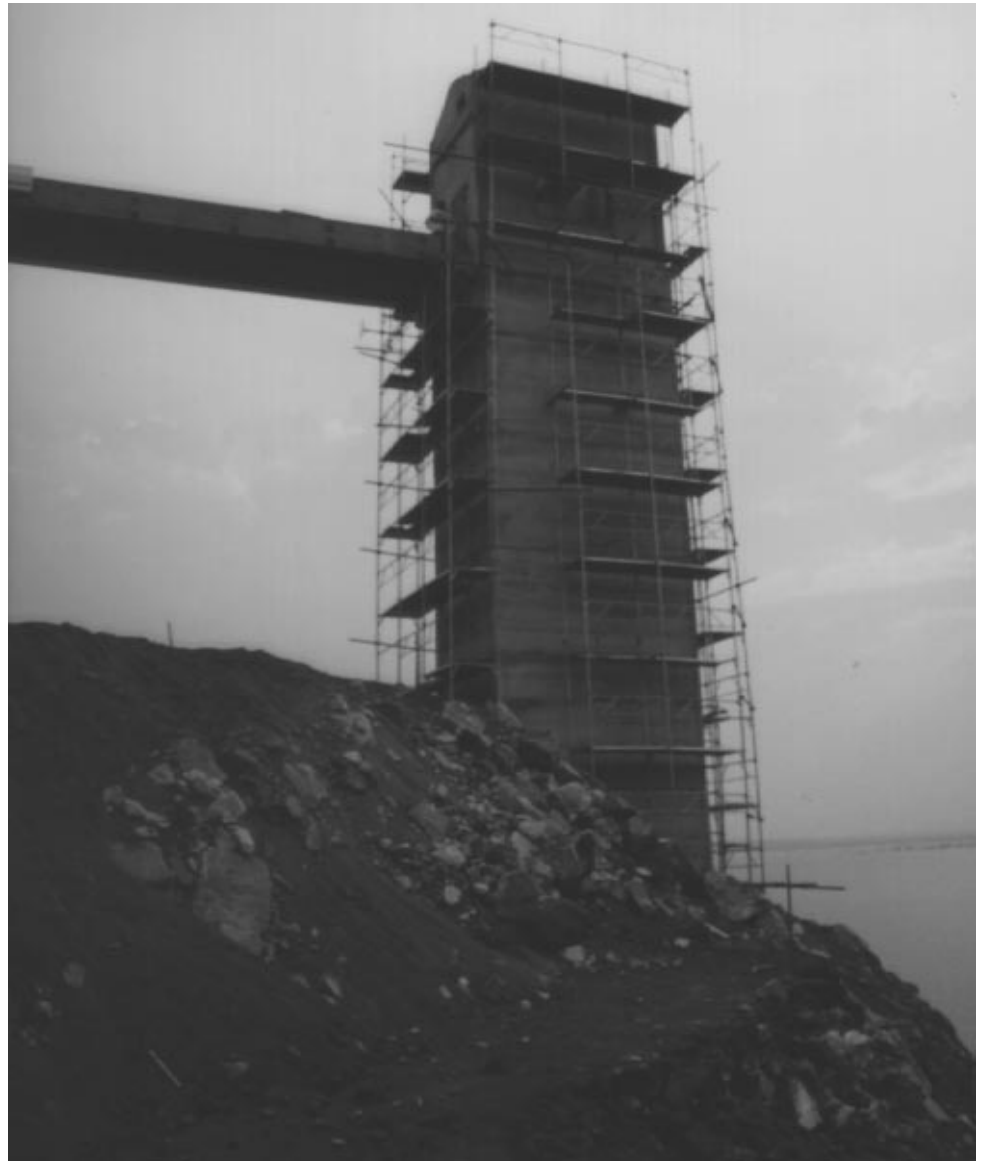
Figure 6: Water Tower in Mozambique That Was Partially Funded as Child Survival
