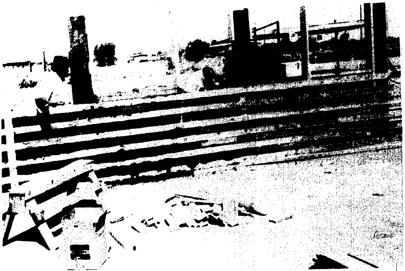
HIP HOUSE BEING BUILT AT THE GILA RIVER RESERVATION BY "IMPROVED SANDWICH" METHOD.
