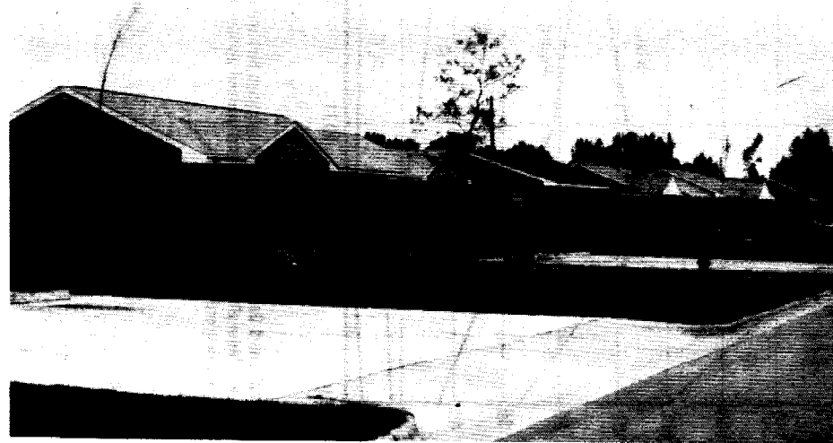
HUD PUBLIC HOUSING PROJECT IN NORTHAMPTON COUNTY, NORTH CAROLINA
