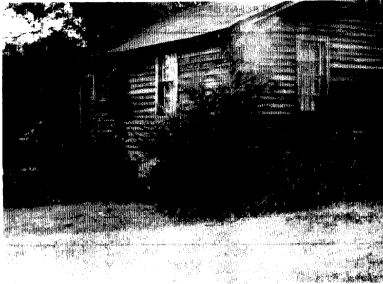
FORMER SUBSTANDARD RESIDENCE OF AN FmHA BORROWER IN CHAMBERS COUNTY, ALABAMA
