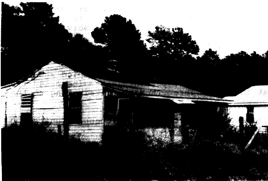
OCCUPIED SUBSTANDARD HOUSE IN NORTHAMPTON COUNTY, NORTH CAROLINA
