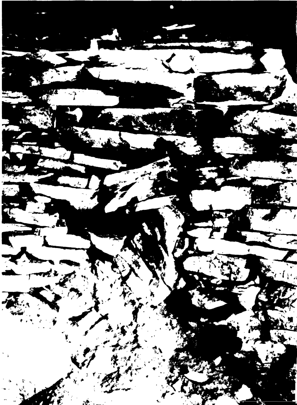
Figure 2.1: Damaged Prehistoric Structure in NPS' Glen Canyon National Recreation Area
