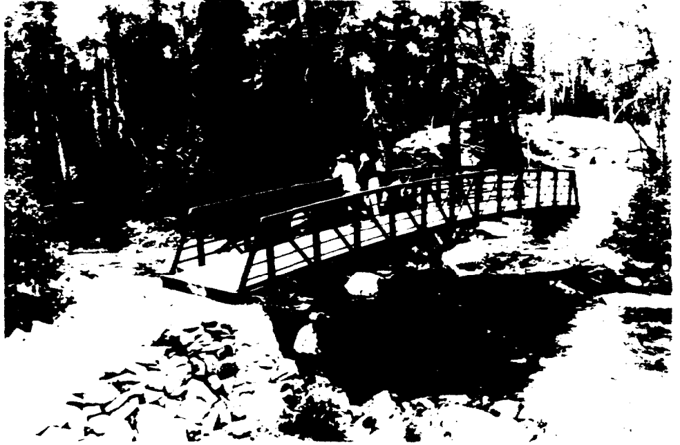
Figure 2.5: Replacement Steel Bridge With Wood Decking, Shoshone National Forest, Wyoming
