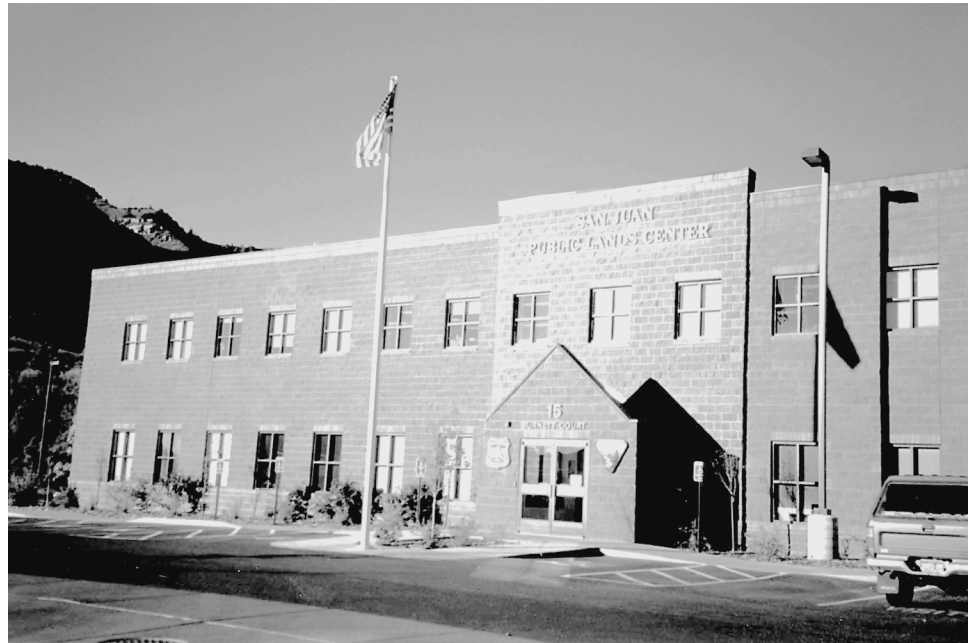
Figure 4: Forest Service and BLM Colocated Unit at Durango, Colorado
