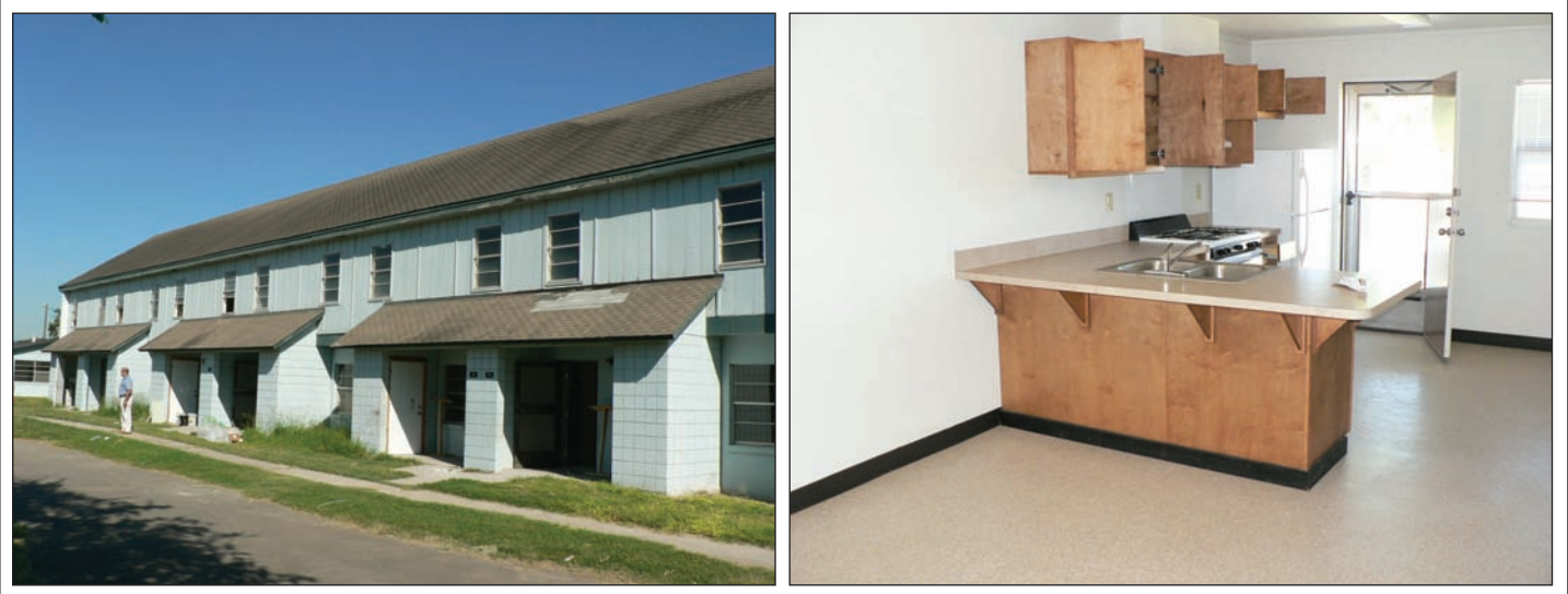
Figure 15: FLH Unit Undergoing Rehabilitation in Texas
