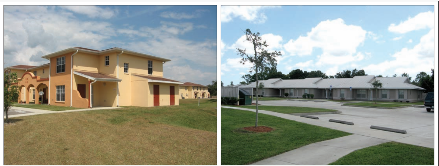
Figure 11: Newly Developed Florida Properties with Low Levels of Disrepair
