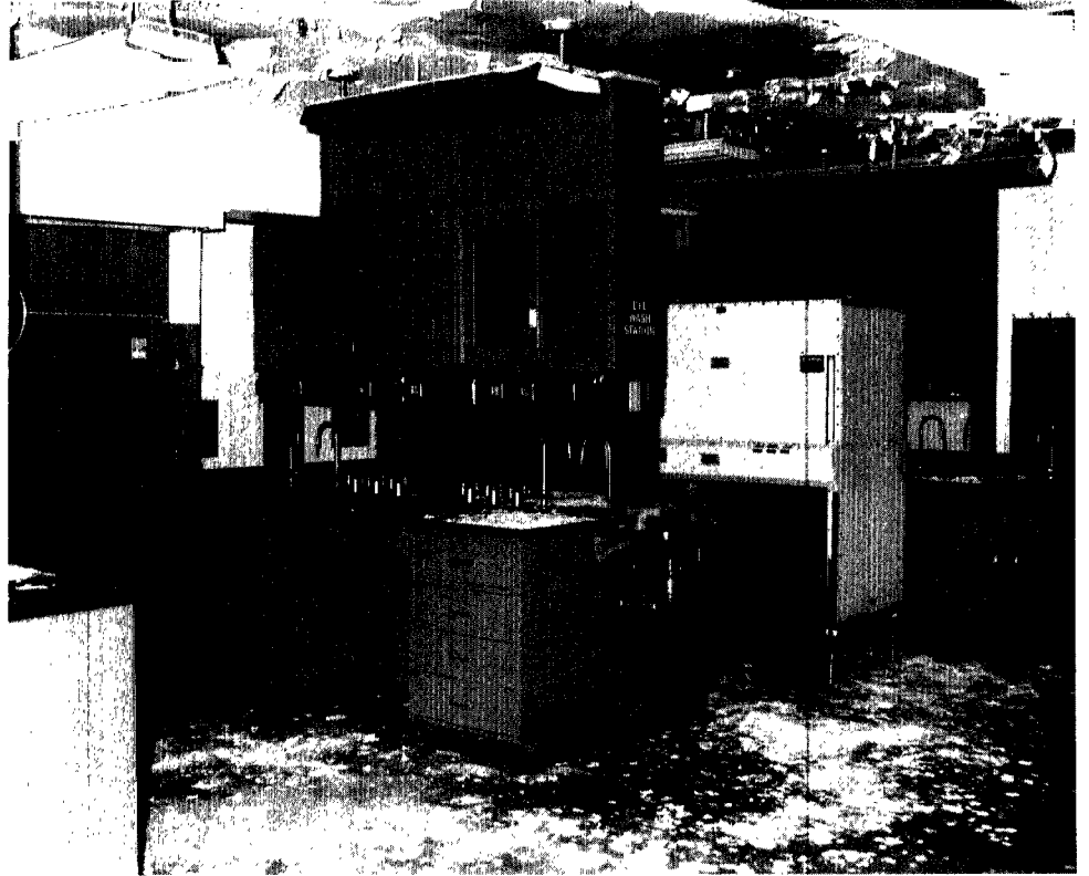
Vacant laboratory scheduled for repair after building's roof is replaced.
