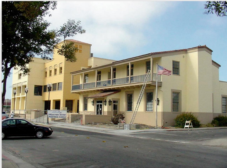
Construction is finishing on the new Cabrillo College campus in downtown Watsonville.
