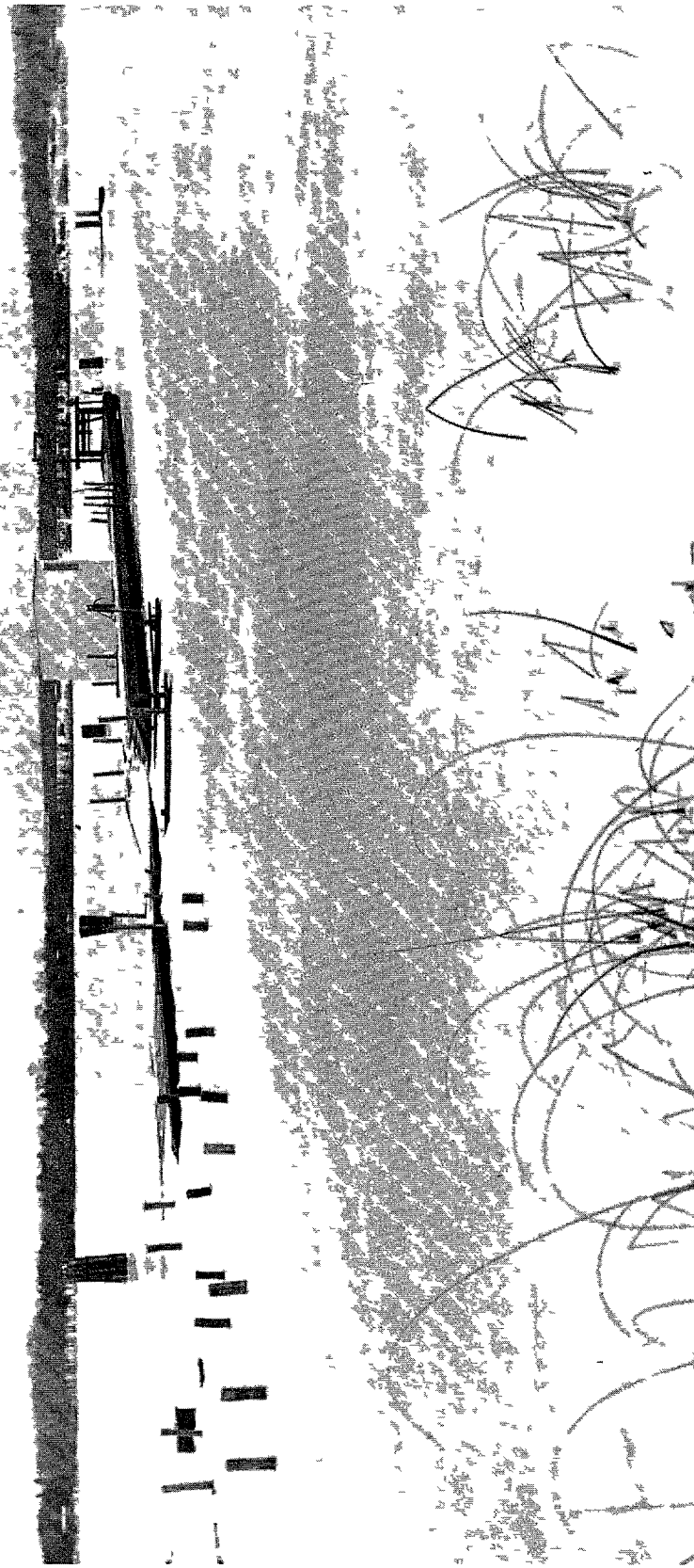
PHOTOGRAPH SHOWING POSSIBLE EFFECT OF LATE NAVIGATION ON SMALL DOCKS - ICE MAY BE LIFTING OUTER END OF DOCK
