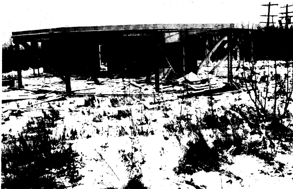
CONTROL BUILDING AT NIKE SITE JIG, 2,038 SQUARE FEET, ORIGINAL COST - $141,000.
