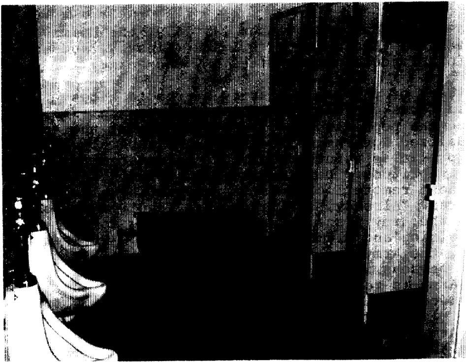
RESTROOM AT PROTECTED NIKE SITE BAY.
