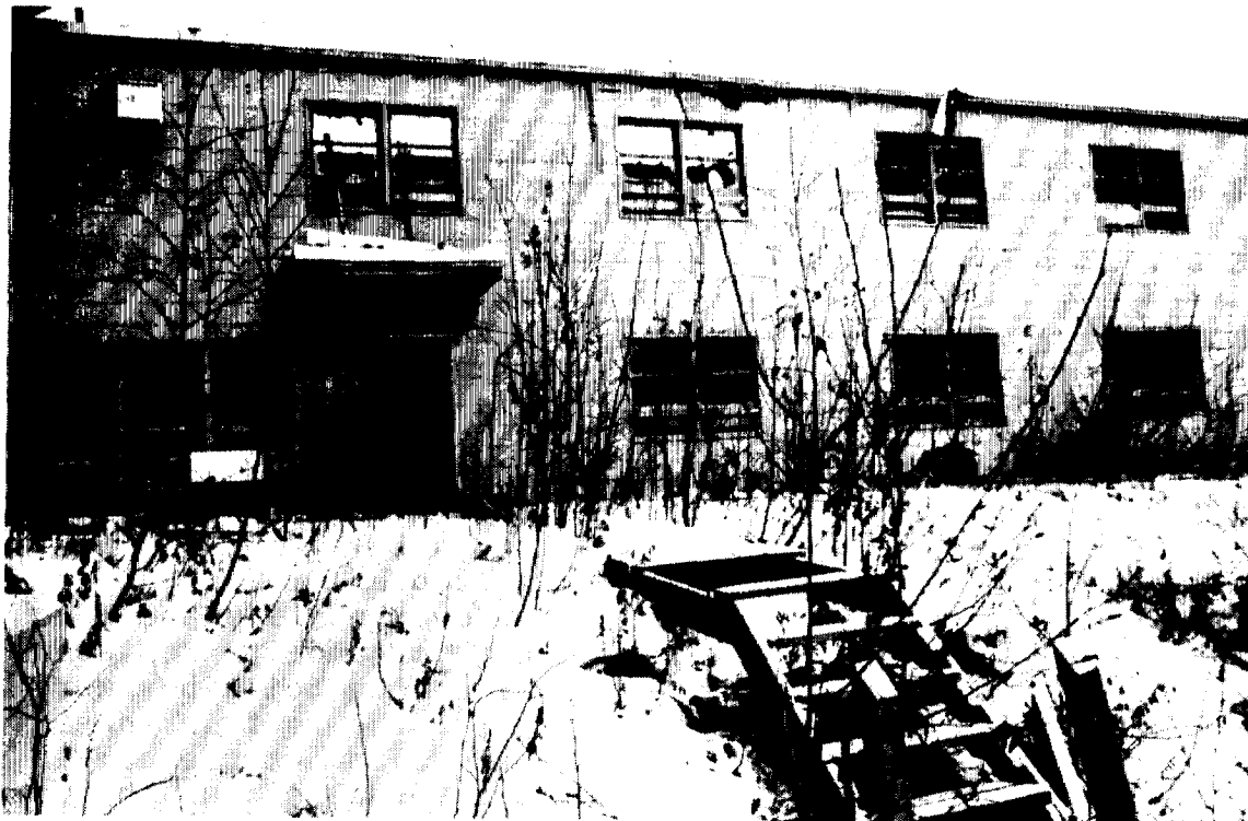
SECTION OF BATTERY CONTROL AND ENLISTED MEN'S BARRACKS, 25,497 SQUARE FEET, ORIGINAL COST - $1,944,500.
