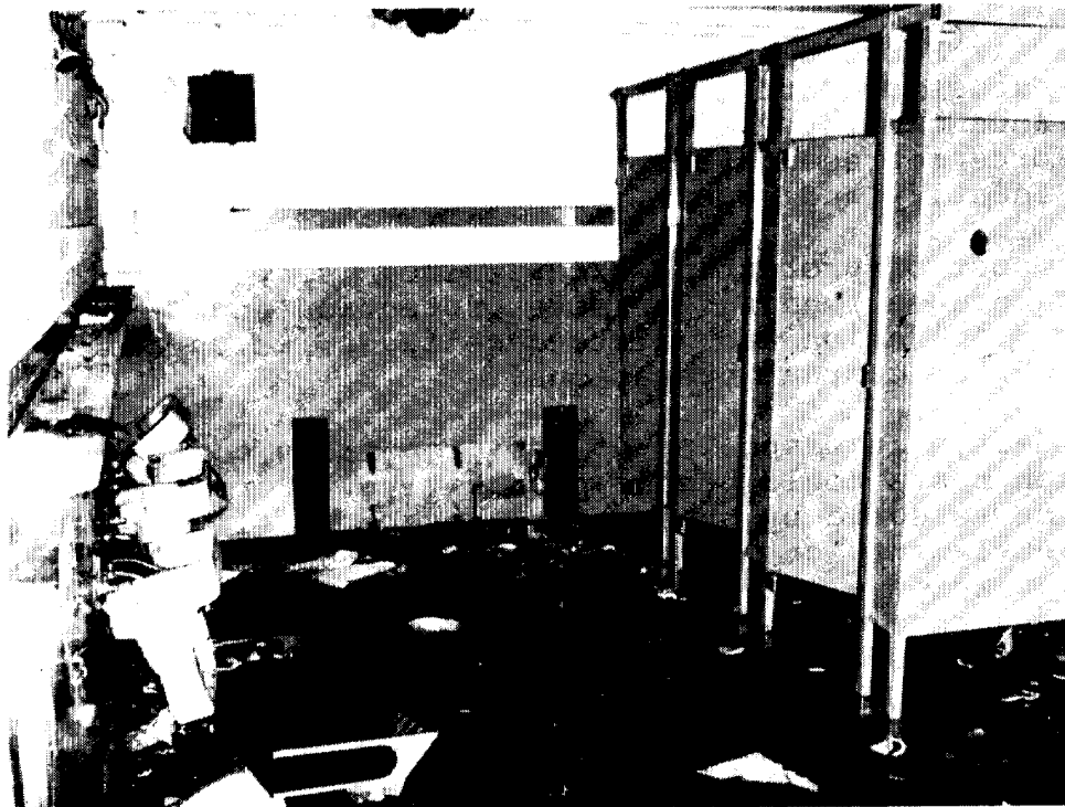
RESTROOM AT UNPROTECTED NIKE SITE JIG.
