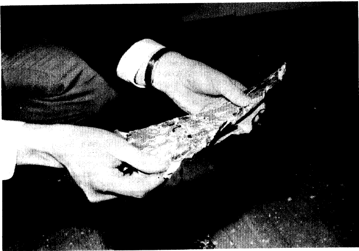
NO INSULATION. THIN MOISTURE BARRIER. FT. EUSTIS
