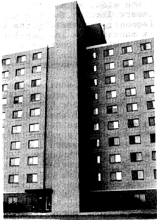
OUTSIDE ELEVATOR INSTALLED USING O&M FUNDS AFTER BUILDING WAS COMPLETED. LANGLEY AIR FORCE BASE
