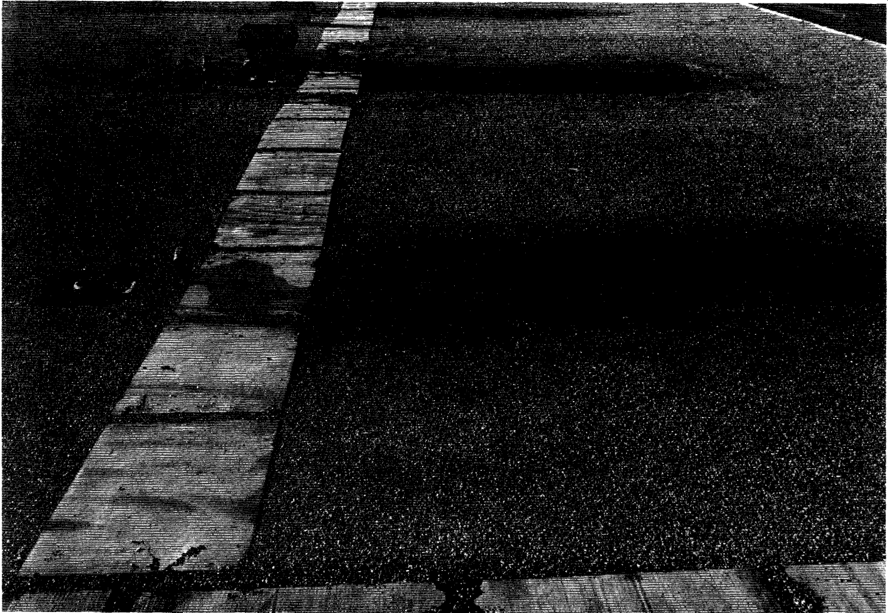
Sagging roof and standing water. Trident training facility, Naval Submarine Base, Bangor, Bremerton, Washington. (U.S. Navy photo.)
