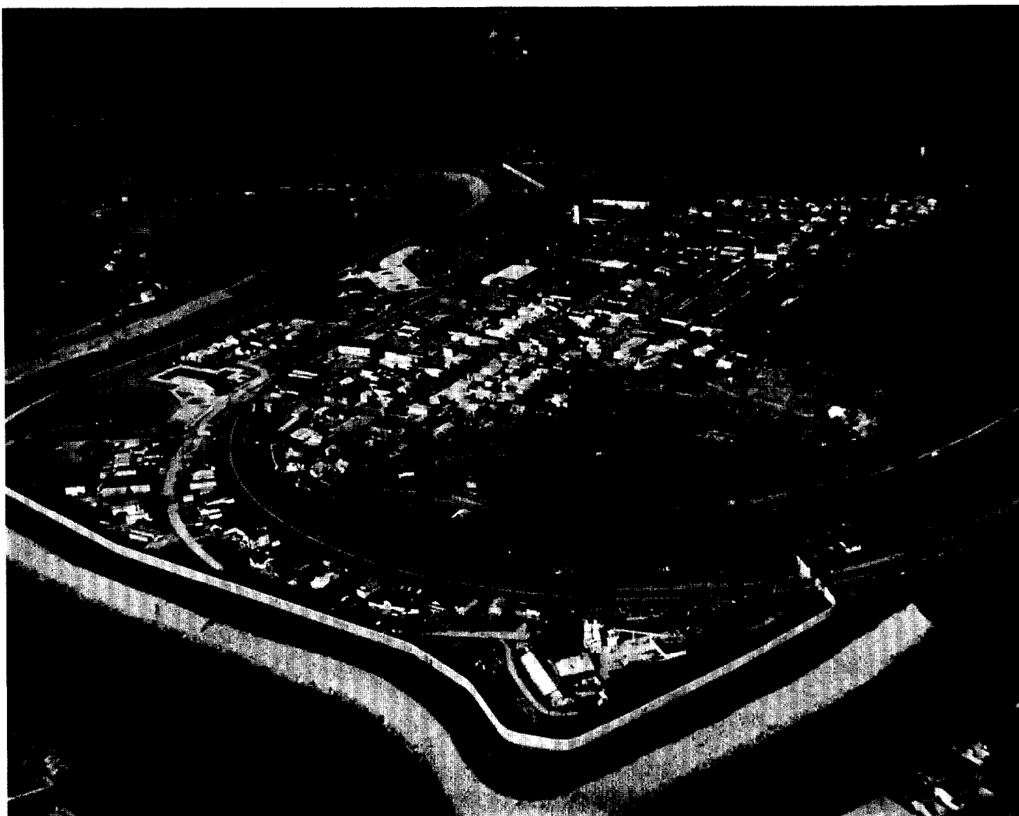
Figure II.3: Nearly Completed Floodwall Atop the Levee
