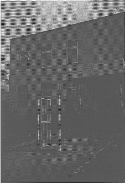
New fence and gate
