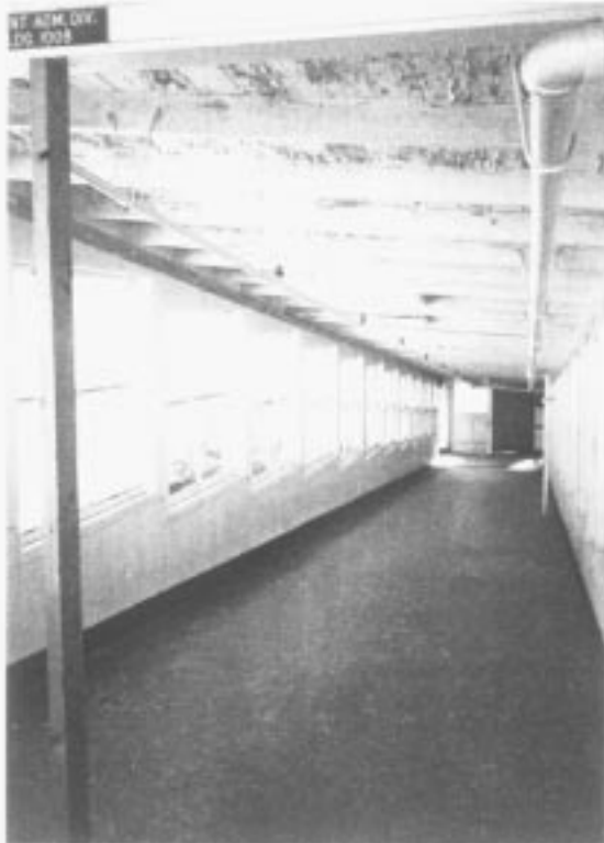
Thoreau Center interior before renovation
