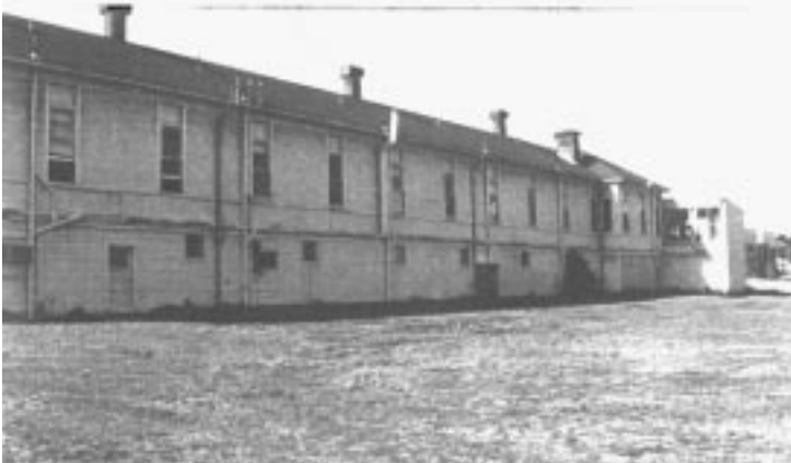
Thoreau Center exterior before renovation
