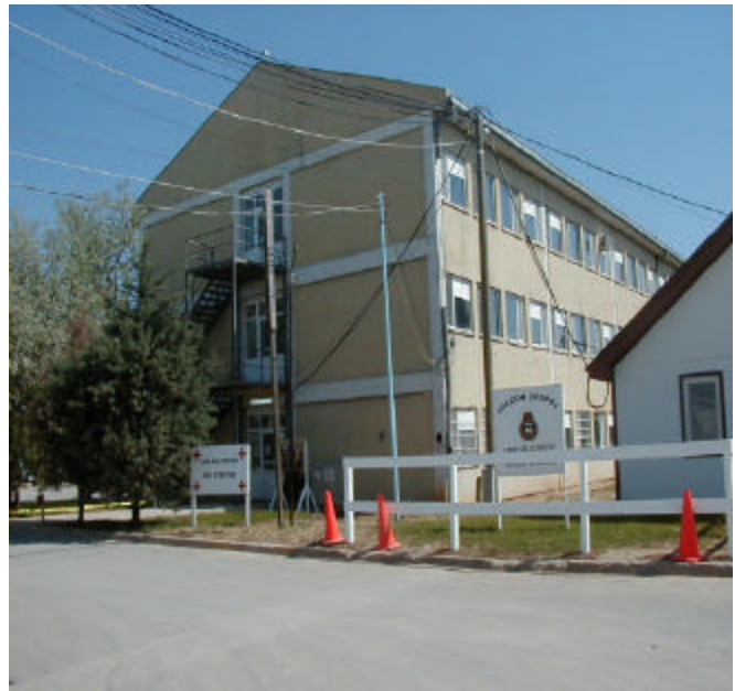
Barracks building, Camp Able Sentry, Macedonia
