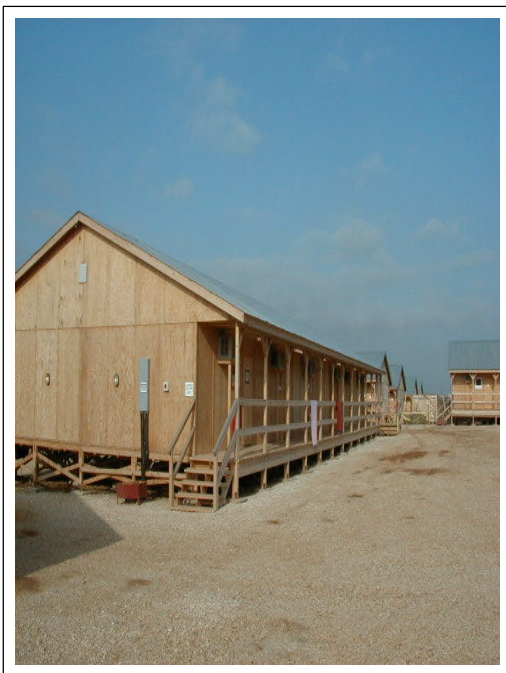
SEAhut at Camp Bondsteel, Kosovo
