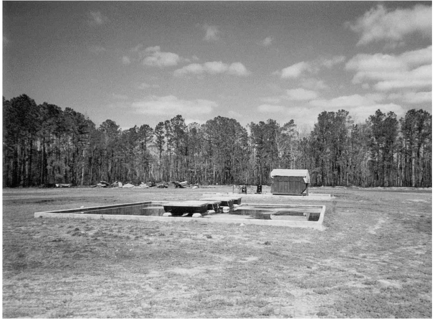
Figure 3: Open Burn/Open Detonation Site
