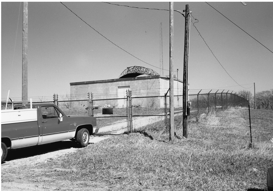
Figure 5: Photo from a Site Visit to a Former Gap Filler Annex
