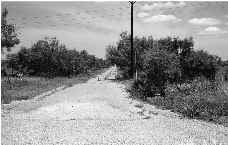
Figure 3: Photo of Locked Gate and Corps Staff Notes from a Site Visit to a 255-Acre Former Nike Missile Site
