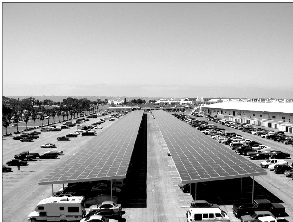
Figure 11: Covered Parking Photovoltaic System at Navy Region Southwest, California
