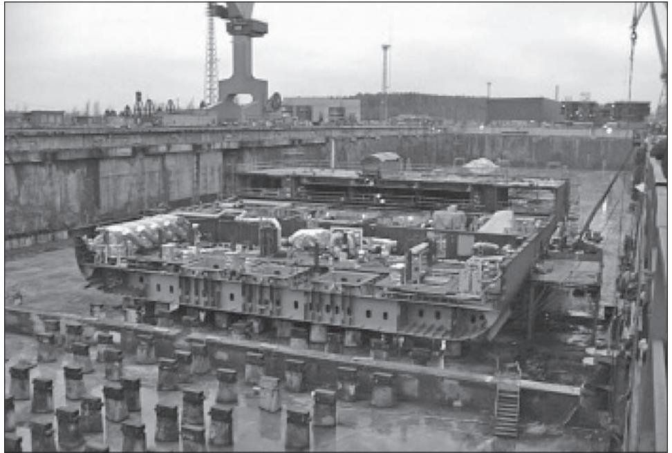
Figure 5: Cruise Ship Blocks in Drydock after Keel Laying
