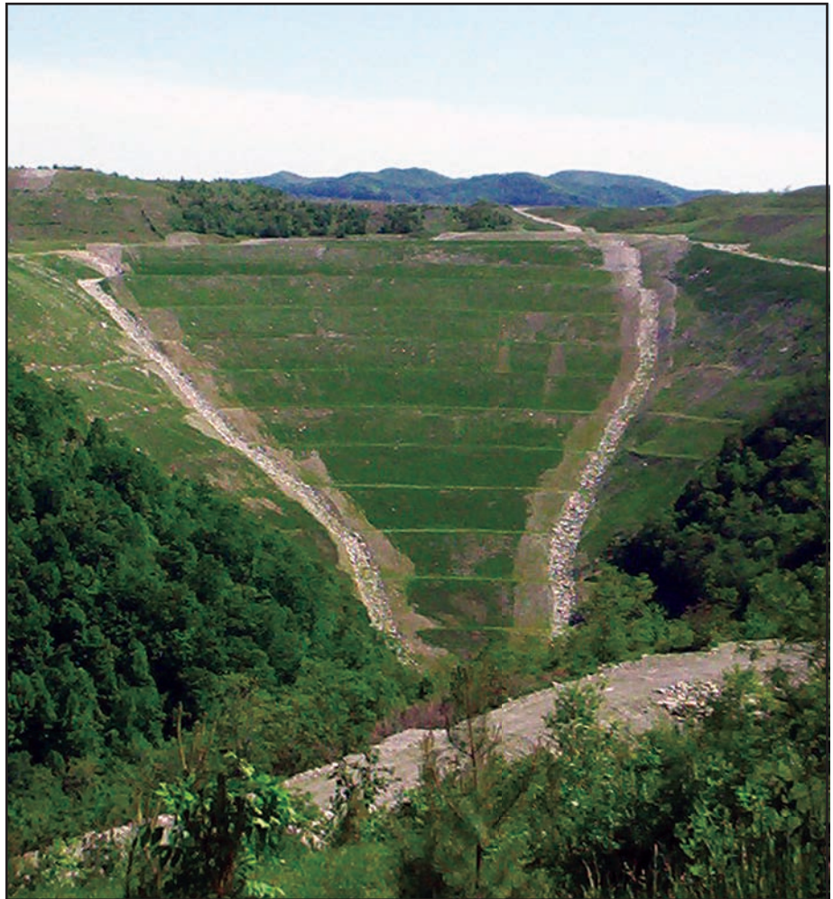
Figure 1: A Valley Fill in West Virginia
