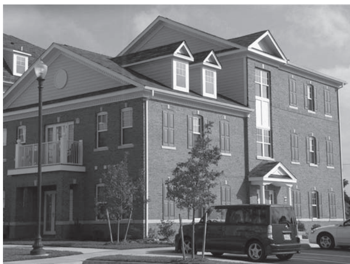
A separate housing unit built with wood-frame construction
