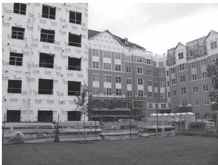
A midrise building being constructed with noncombustible materials
