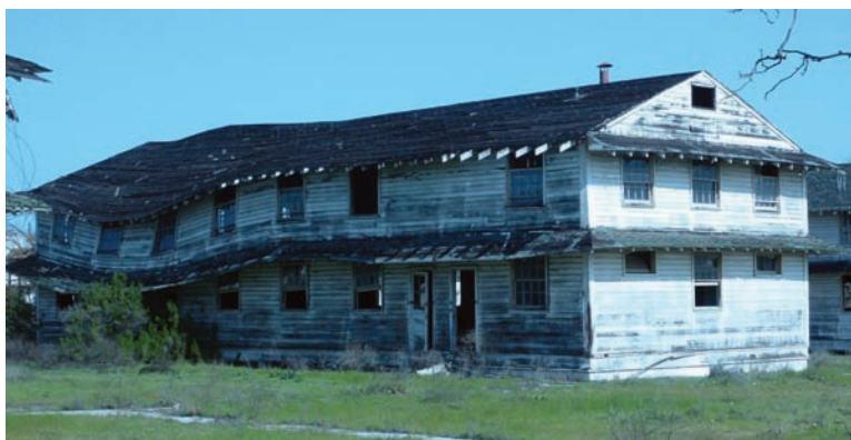
Excess World War II-Era condemned building
