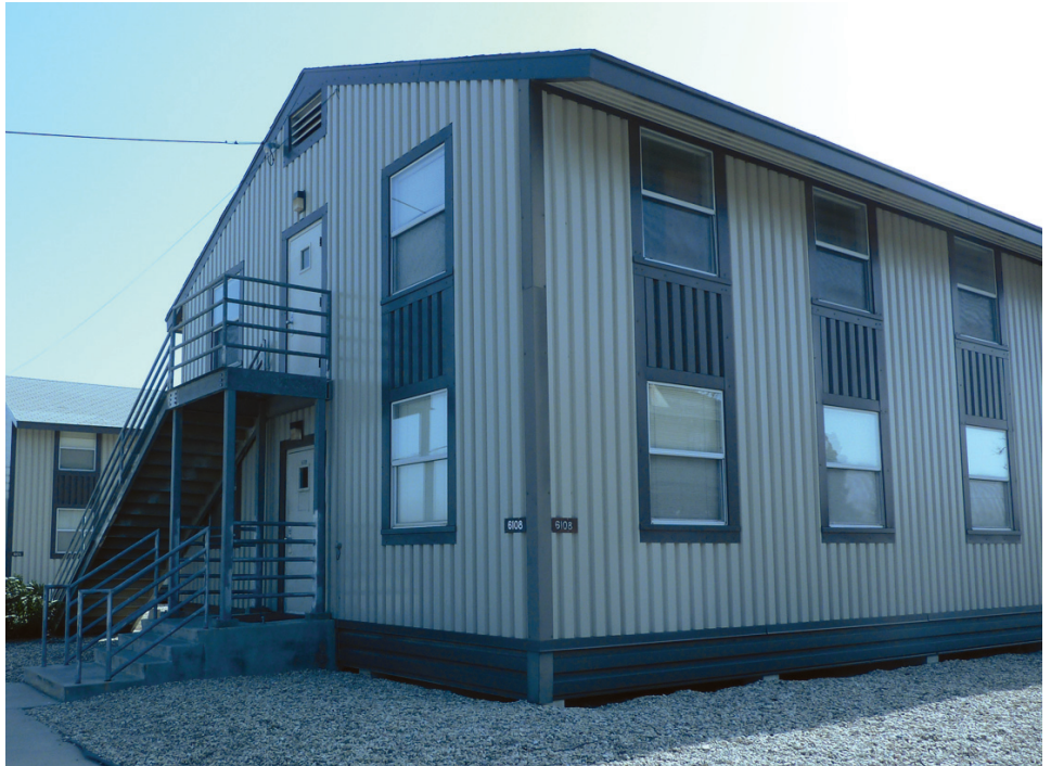
Figure 11: Renovated Temporary World War II-Era Building at Camp Roberts
