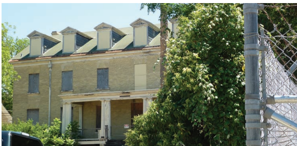
Figure 7: Building 189—the Nurses' Quarters—Next to the Installation Borders at Fort Sam Houston
