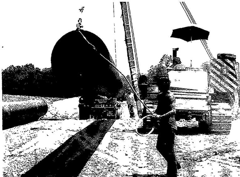
A DITCH IS EXCAVATED TO AN APPROPRIATE DEPTH AND WIDTH. JOINTS OF PIPE (40 , 60 , OR 80' IN LENGTH) ARE HAULED TO THE RIGHT OF WAY AND STRUNG ALONG THE DITCH.
