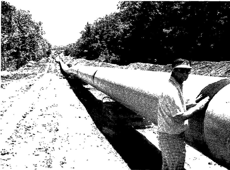
THE PIPE IS COATED WITH PROTECTIVE MATERIALS EITHER "OVER THE DITCH" OR AT A SITE REMOVED FROM THE CONSTRUCTION AREA. PIPE COATINGS ARE INSPECTED AND TESTED.
