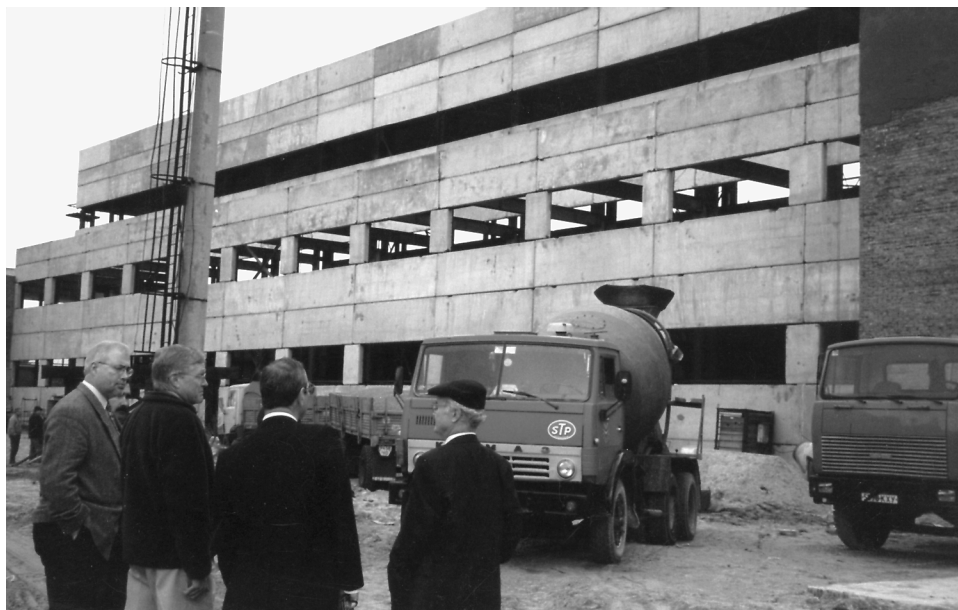
Figure 10: Status of Construction of the Chernobyl Heat Plant, as of October 1999
