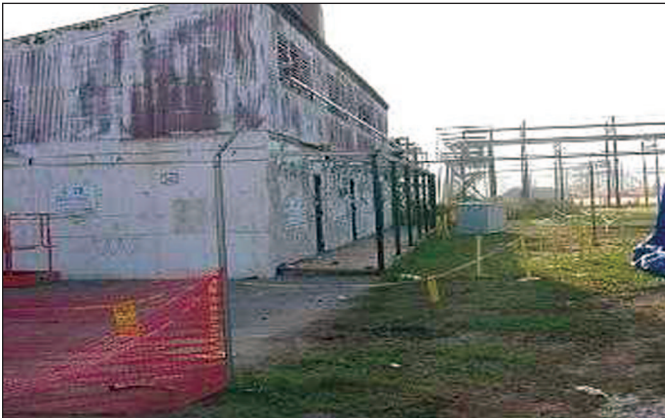
Before D&D. Fluorine storage facility at the Oak Ridge plant. Fluorine gas is a key component in the uranium enrichment process.
