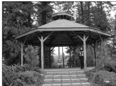
Kiosk Constructed from Small-Diameter Wood
