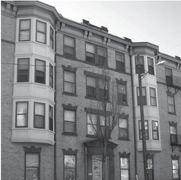
Side view of Greystone Apartments exterior.
