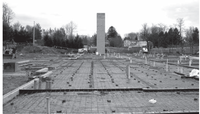
The concrete slab for two new buildings at Hopewell Courtyard.
