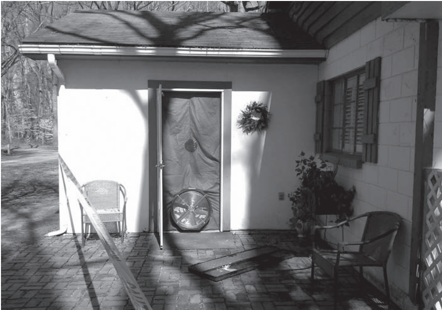
Outside view of blower door set-up
