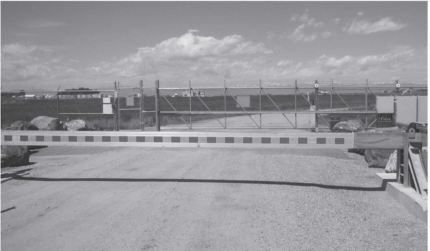
Figure 5: Antiterrorism Crash Barrier Gate Installed inside Fenced Perimeter of a Critical Facility
