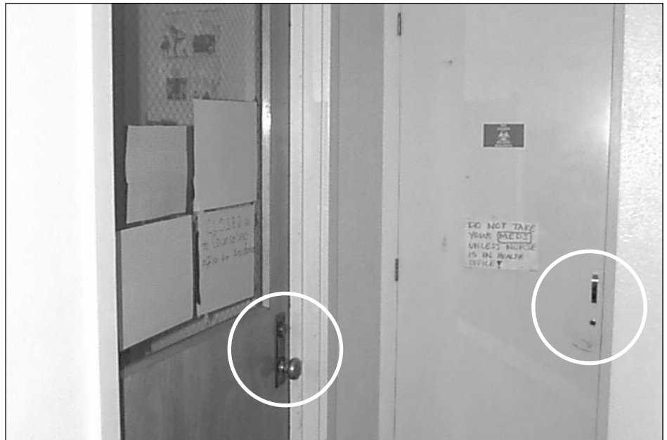
Cabinet and door locks school B
