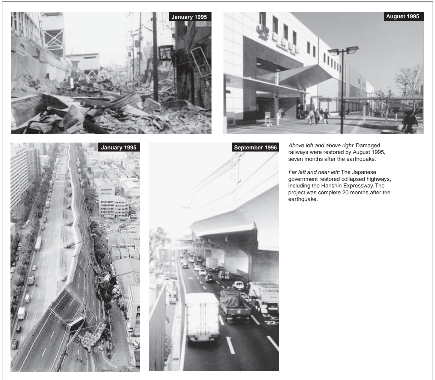
Figure 14: Japan Restored Damaged Railways and Highways Approximately 20 Months after the Earthquake
