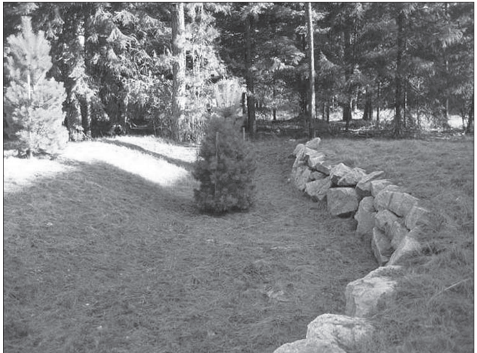
Figure 2: View of Antivehicle Barriers Created to Help Secure a Courthouse
