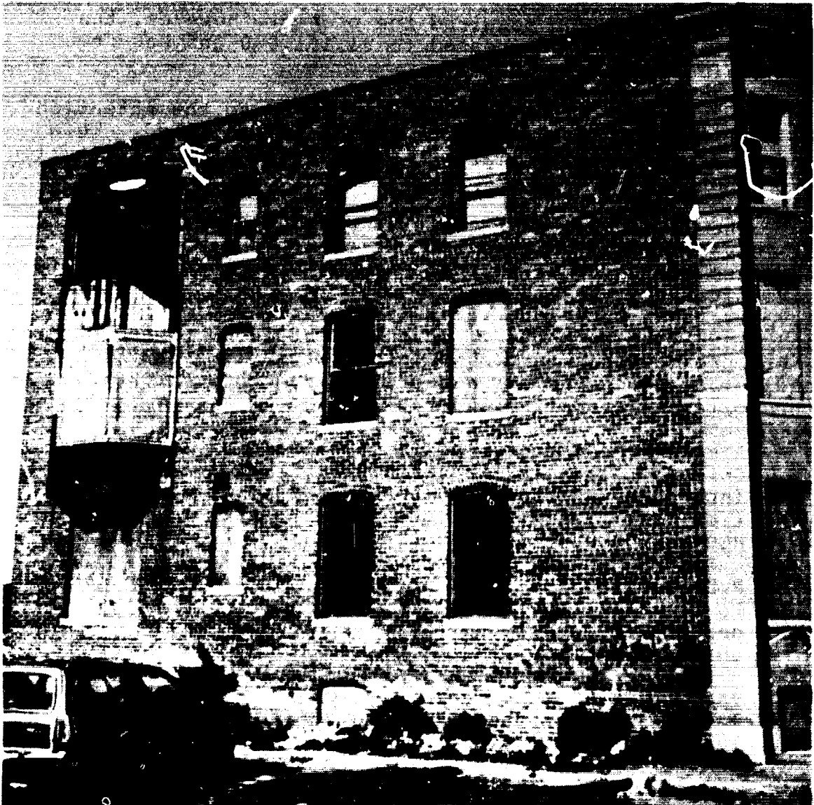
Side view showing missing and partially boarded windows.
