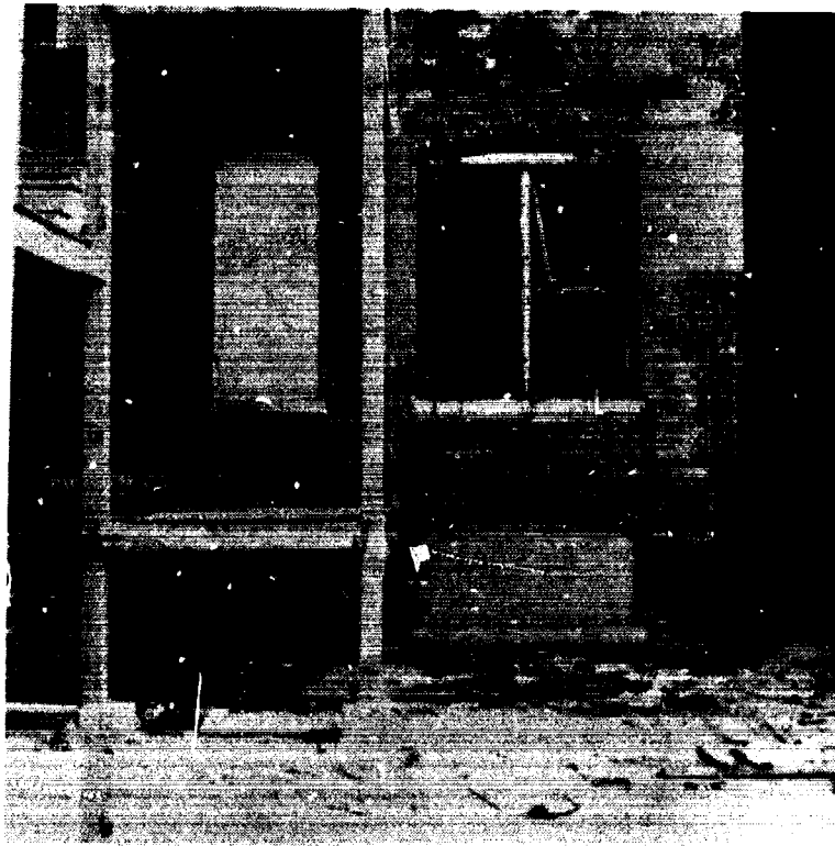
Rear view showing missing window and door.
