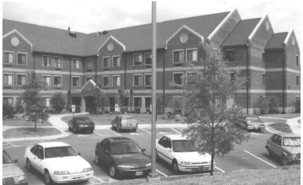
Figure I.6: Assembly Terrace Section 202 Project, Winston-Salem, North Carolina
