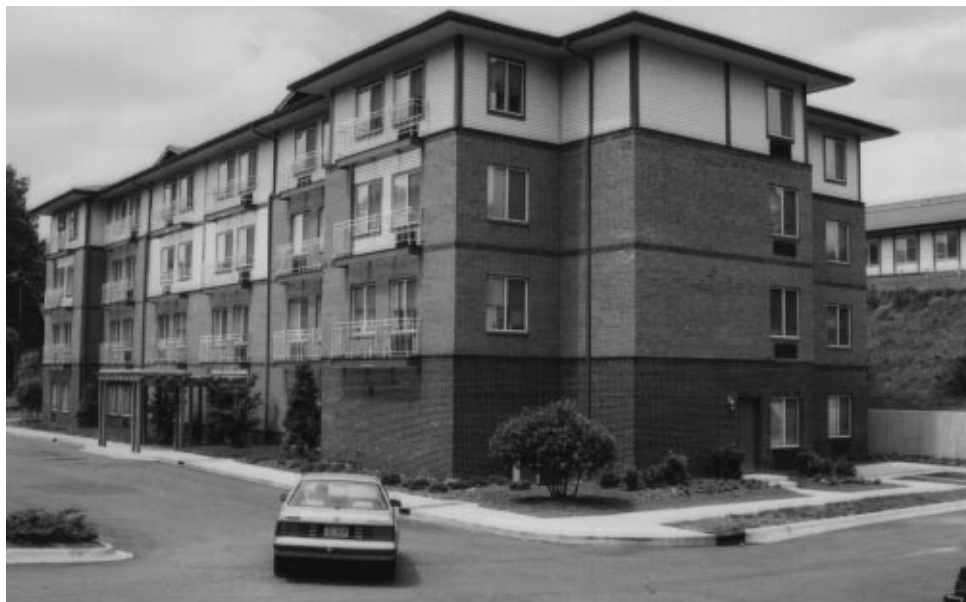
Figure I.5: Granville Plaza Section 202 Project, Winston-Salem, North Carolina
