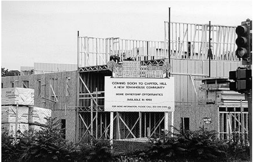
Figure II.10: New Construction at Ellen Wilson
