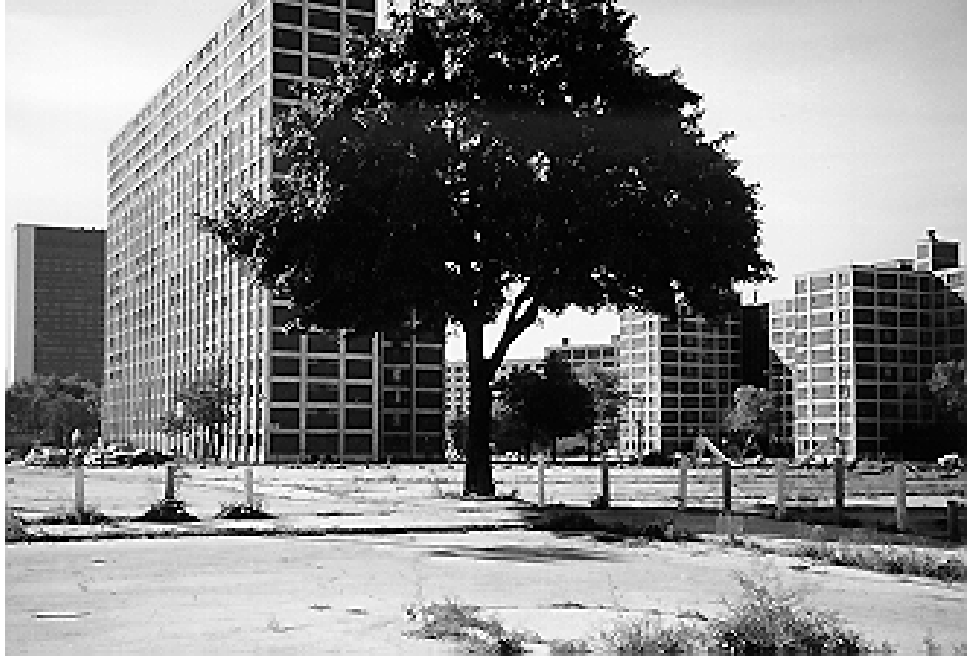
Figure II.12: High-Rise Buildings Awaiting Demolition at Cabrini Homes Extension
