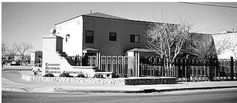
Completed section near entrance, including the new wrought iron fencing
