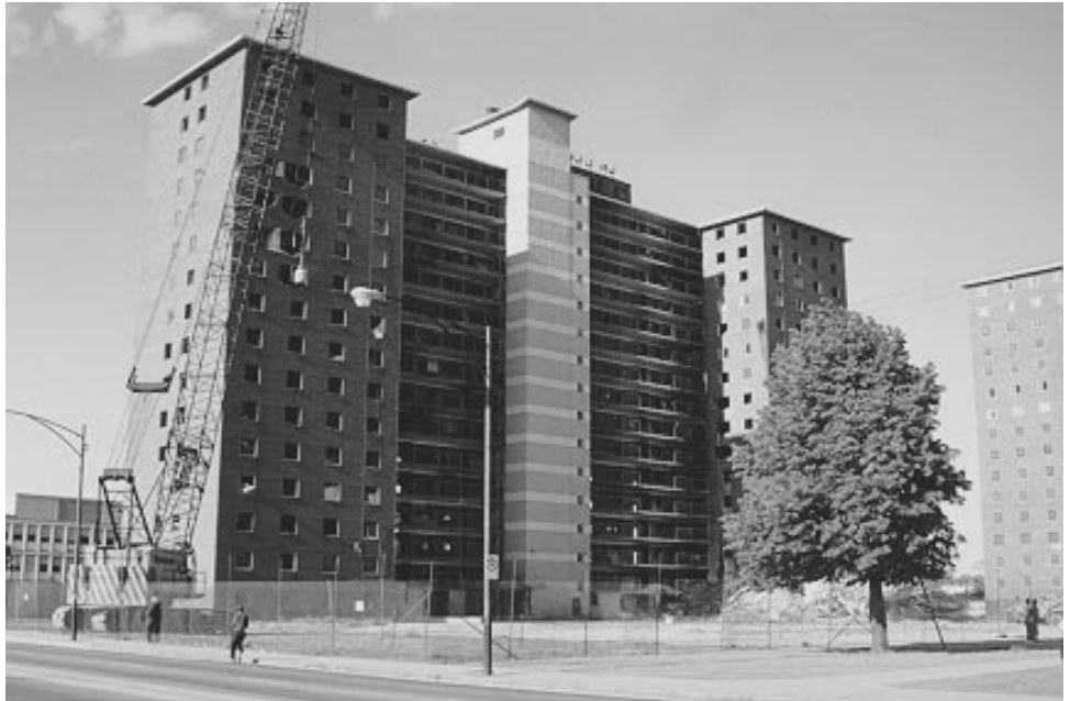
Demolition begins at Robert Taylor B, May 18, 1998
