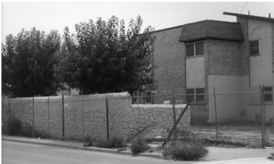
Before renovation with remnants of stonewall standing
