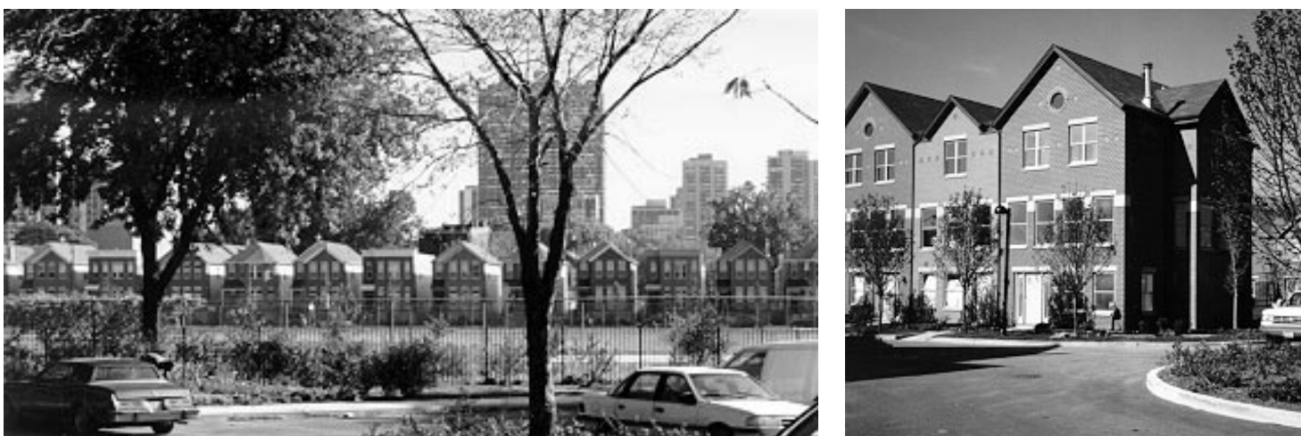
Figure 4: Construction Adjacent to Cabrini Homes Extension, Chicago, Illinois
