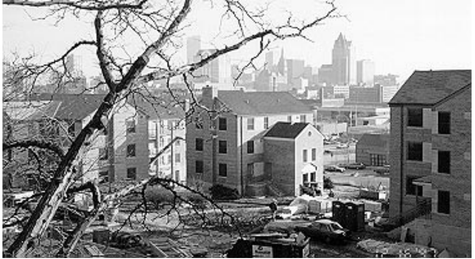
Rehabilitated units under construction
