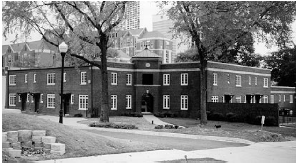
Rehabilitated historic building
