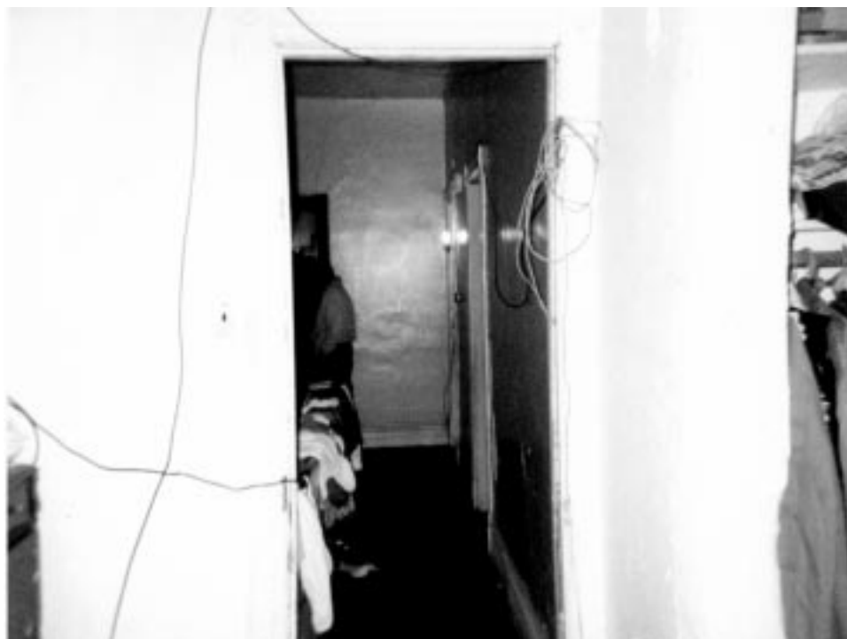
Figure 9: Electrical Wiring Strung Along Outside of Wall Instead of Inside the Wall
