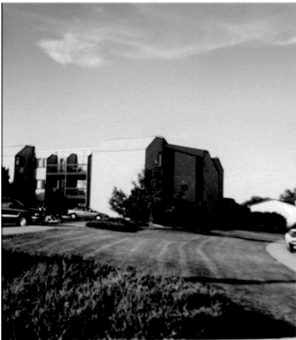
Figure 7: Photograph of Parkside Apartments
