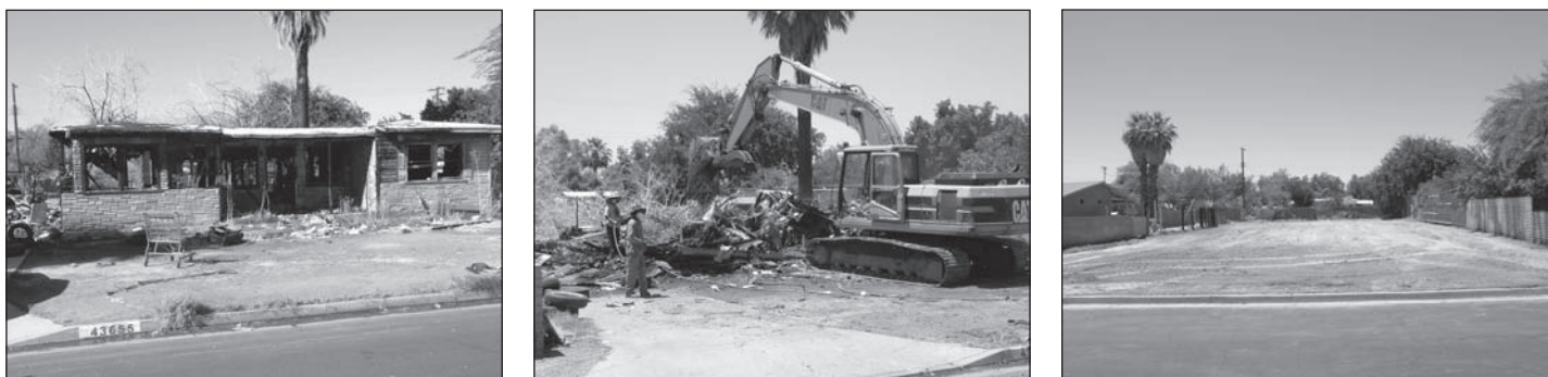
Figure 11: Demolition of a Single-family Property in Indio, California
