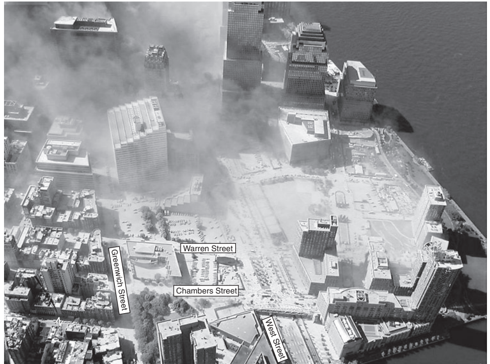
Figure 2: Collapsed WTC Towers on September 11, 2001
