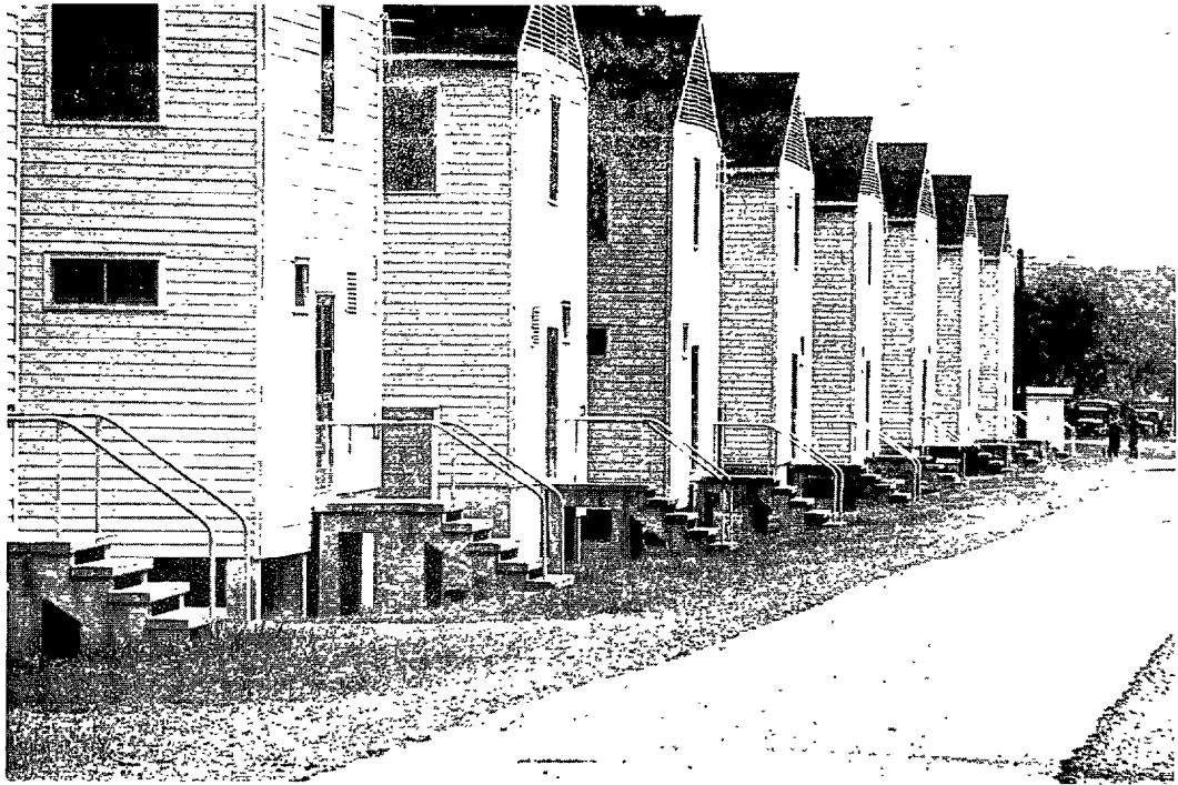
FORT CHAFFEE: BARRACKS USED FOR HOUSING REFUGEES.
