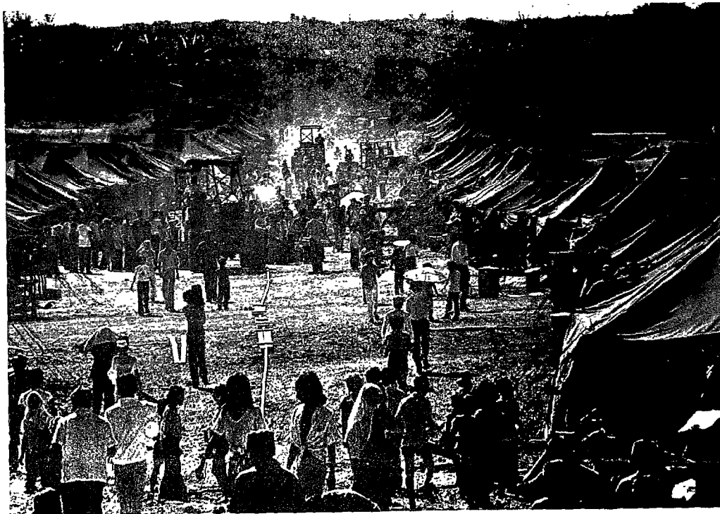
GUAM: CONSTRUCTION IN PROGRESS WHILE REFUGEES ARRIVE. Official U.S. Navy Photograph
