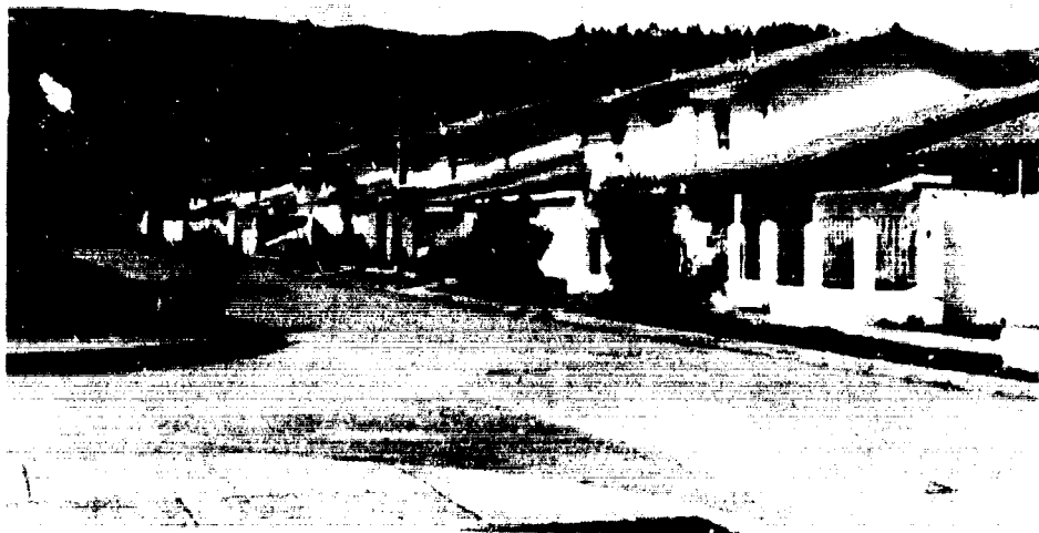
IDB RECONSTRUCTION HOUSING PROJECT IN PERU.
