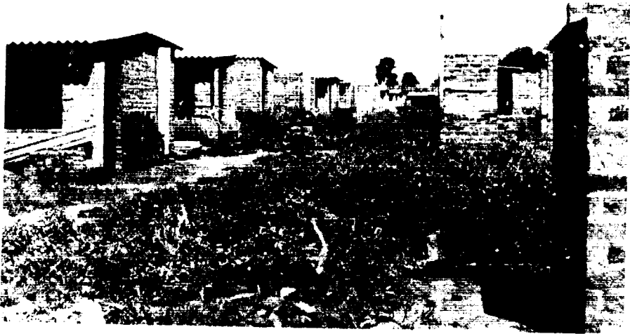
HOUSING UNITS UNDER CONSTRUCTION IN SONSONATE, EL SALVADOR, AS PART OF THE WORLD BANK/FOUNDATION FOR MINIMUM HOUSING SITES AND SERVICES PROJECT.
