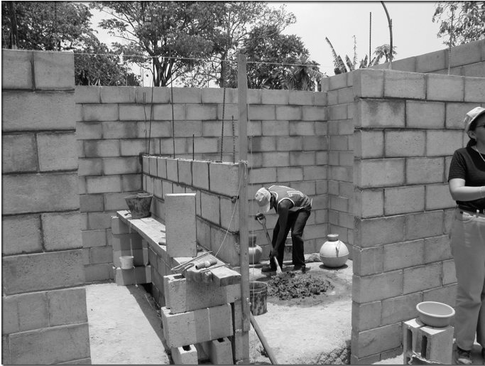
Figure 4: Houses under Construction, Being Inspected, and Completed
