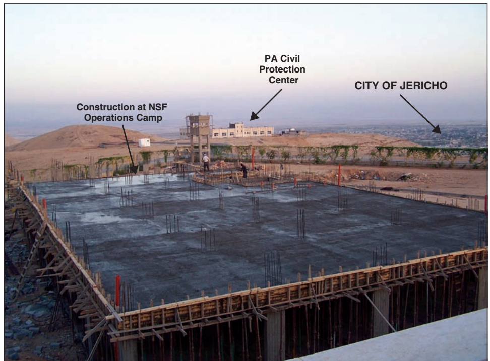
Figure 7: U.S. Funded Construction at the NSF Operations Camp Near Jericho
