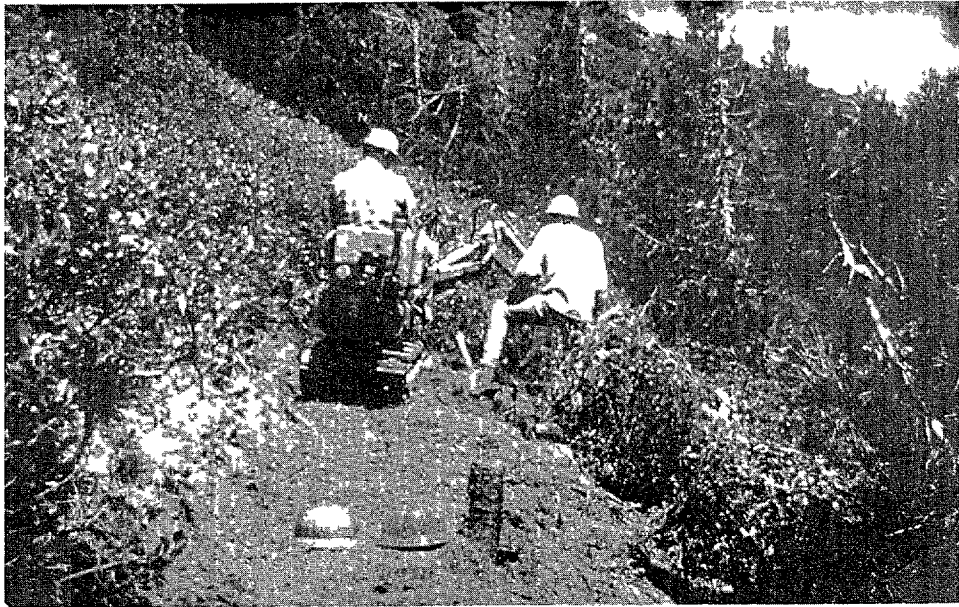
Photo 5: Trail machine developed specifically for the construction of trails.
