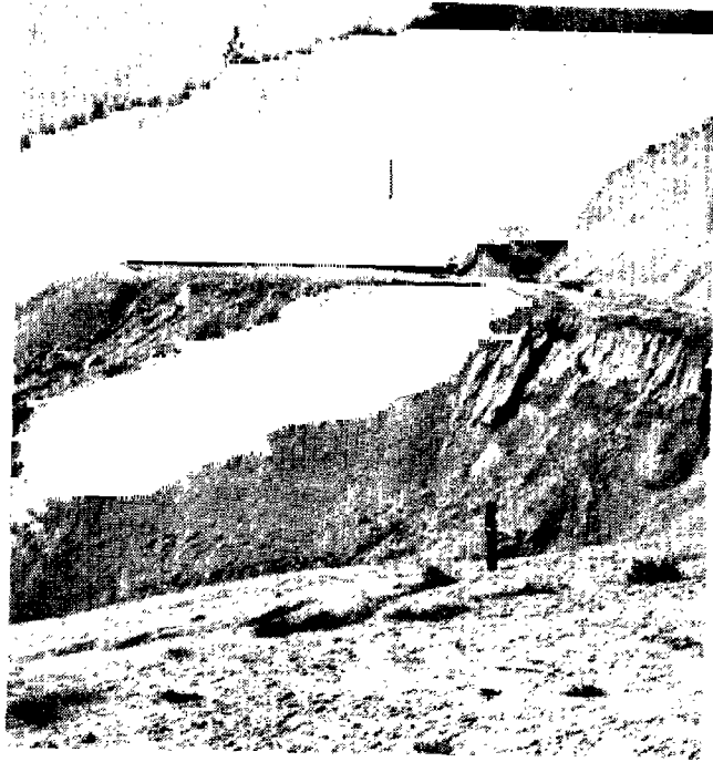
EROSION PROBLEM CAUSED THROUGH SUBDIVISION IN YOSEMITE NATIONAL PARK
