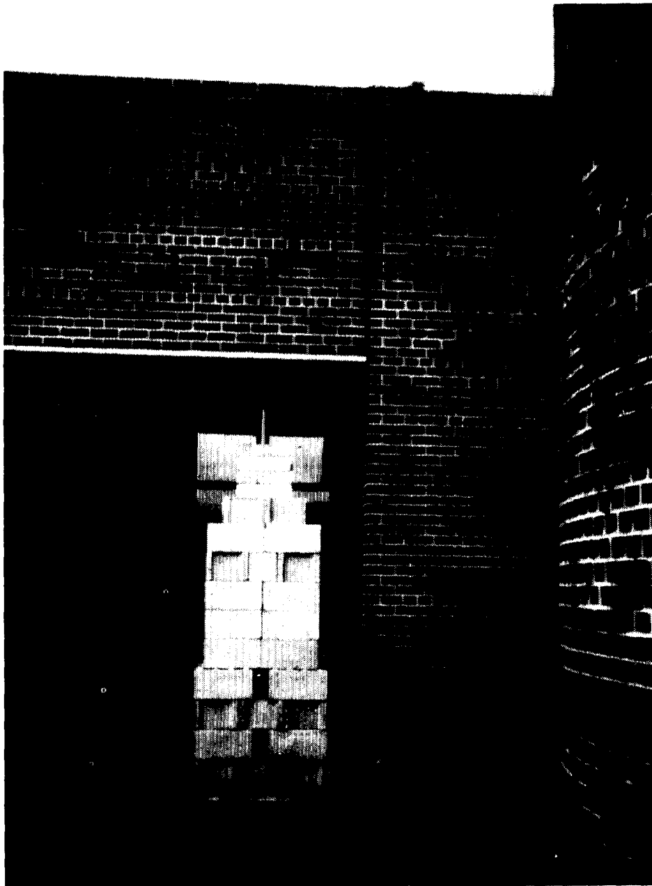
FIG. 10 ADJUSTABLE PROP INSTALLED AT ELEMENTARY SCHOOL BELLE VERNON, PENNSYLVANIA
