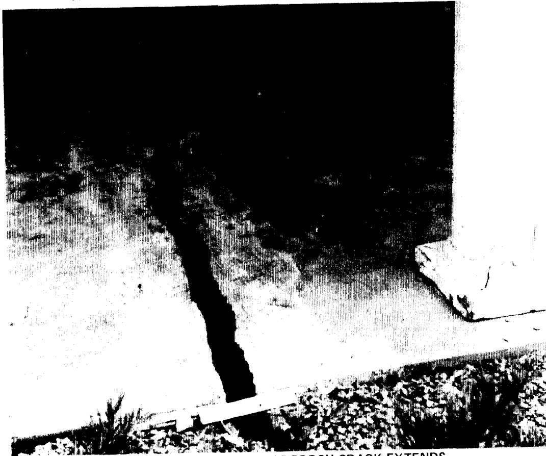
FIG. 5 EXTERIOR CONCRETE PORCH CRACK EXTENDS THROUGH BASEMENT FOUNDATION WALLS
