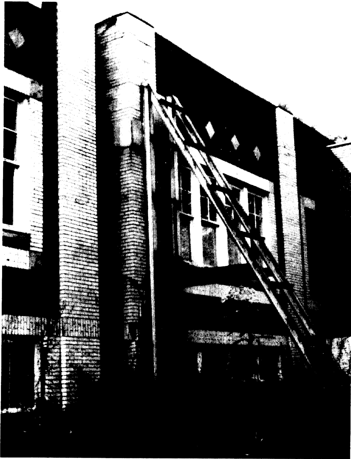
FIG. 12 DAMAGED AND ABANDONED HIGH SCHOOL BUILDING WITH EXTERIOR STEEL SUPPORT BRACING FARMINGTON, WEST VIRGINIA
