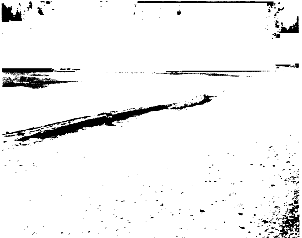
Figure 5.9: Raised Wave of Asphalt in the Center of a Yellowstone National Park Road, Wyoming
