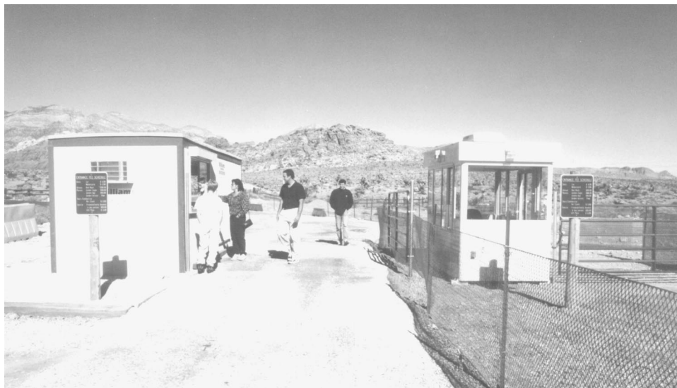
Figure 2.3: New Entrance Station Under Construction at Red Rock Canyon—a BLM Demonstration Site in Nevada
