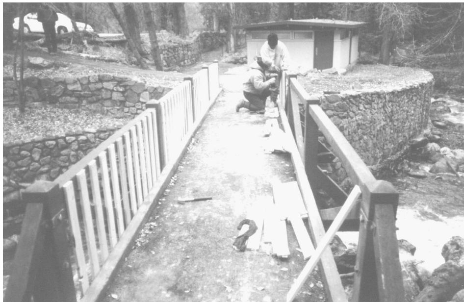
Figure 4.2: Bridge Rehabilitation in Popular Picnic Area at American Fork Canyon, Utah
